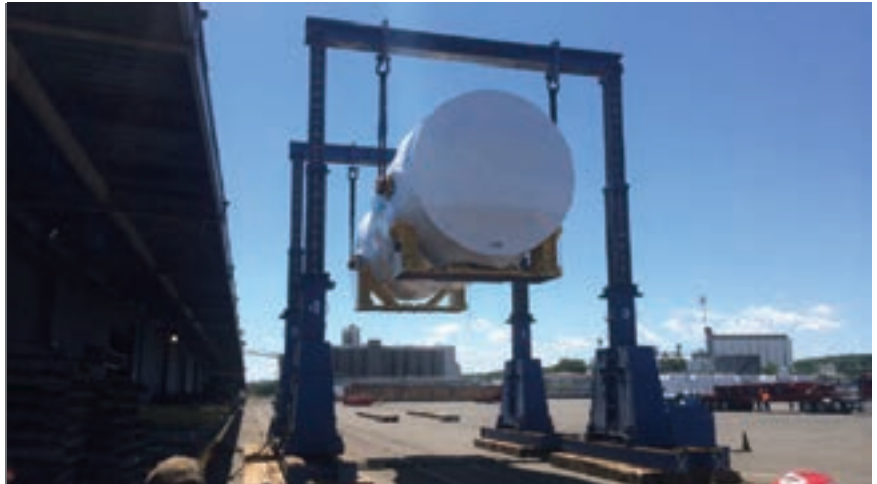
The speedy delivery of critical components keeps power plant construction project on schedule.
