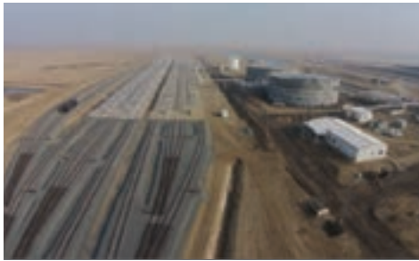
Grassroots crude oil rail car (aerial view) unloading facility was completed in late 2014 with zero recordable injuries and zero lost time accidents.
