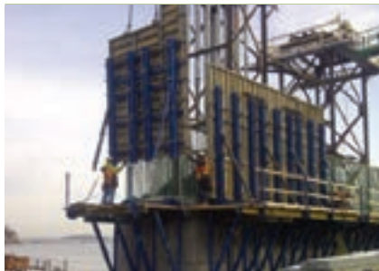
Fore River Bridge Quincy, Mass. | Completion: Dec. 2017
