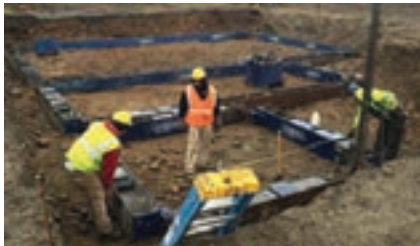
Mabey Inc. power brace system readied for sheet and frame shoring system
