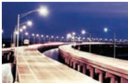
The award-winning Volkert-designed Jubilee Parkway (Bayway) bridge carries I-10 over Mobile Bay.
