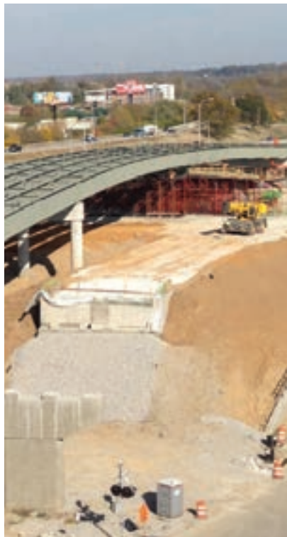
Gamco Scaffold Shoring sets the foundation for safe, efficient bridge construction.
