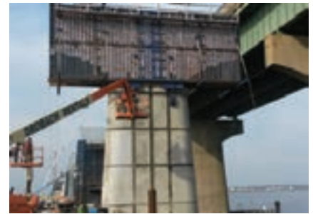
Doka's steel girders span large distances without any additional support or shoring.
