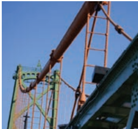
Angus L. Macdonald Bridge, Halifax, Nova Scotia
