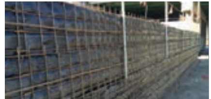
U.S. 6 Over Garrison Street Bridge Denver, Colo.
